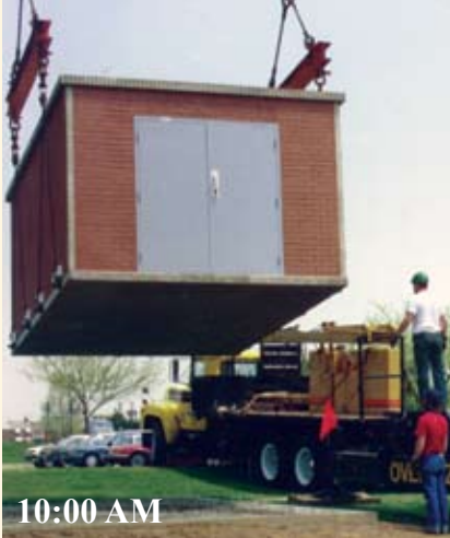
Simple site preparation, no footings required
