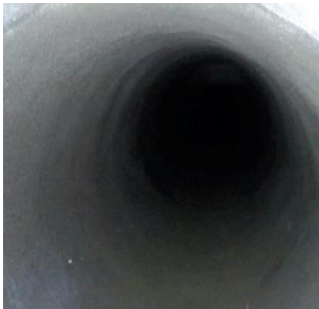
Spray applied 1.75" thickness.
