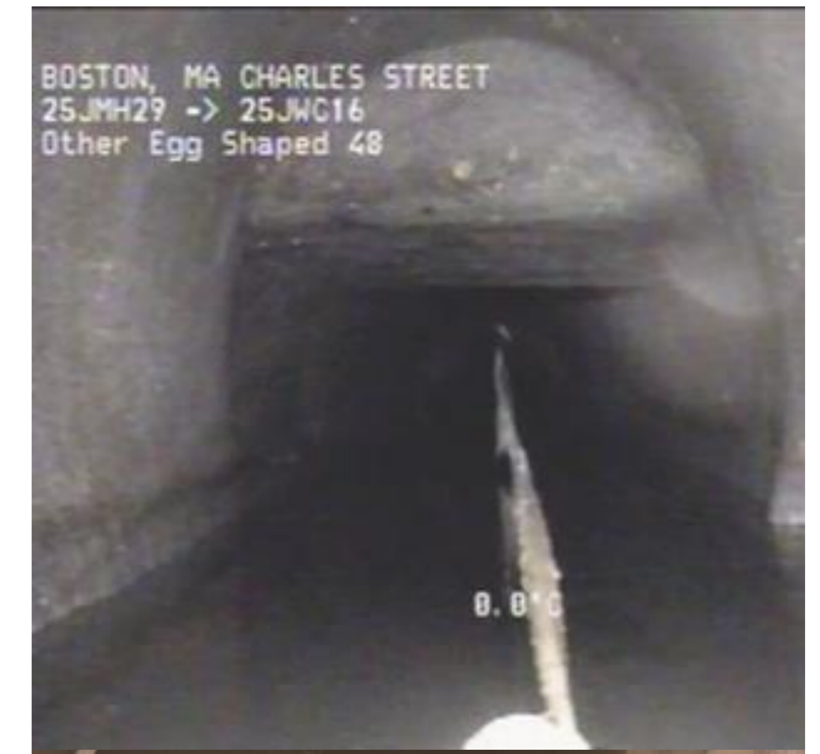
CCTV Camera inspection conducted at one year by owner.
