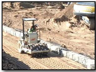
At times, a **filter fabric** may be specified behind the drainage aggregate material. This helps keep the drainage zone clean and free from sedimentation. If present, wrap the fabric forward over the drainage aggregate as the other backfill material is placed.
