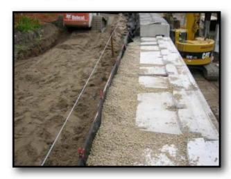
When **drain tile** is used, it should be located as shown in the plans or drawings. Generally, the drain tile runs along the back of the wall and is at the bottom of the drainage aggregate zone at an elevation at or above the bottom finished grade level. Drain tile should "daylight" at least every 50' along the length as well as at every low point in the wall.
